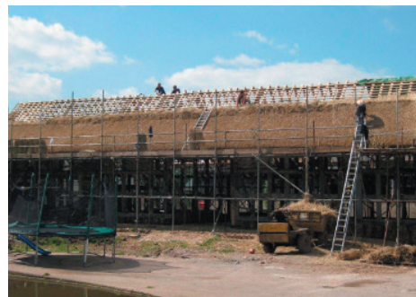
Straw barn in progress nr Tenbury for Natural England by Keith Walden
