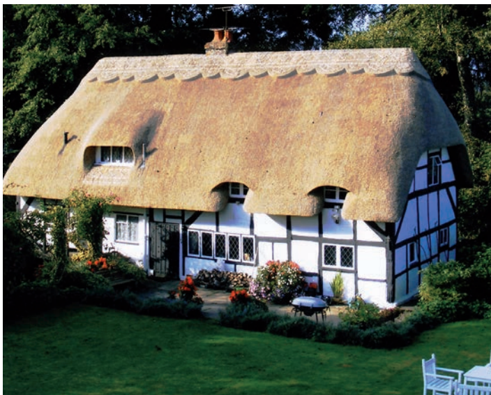
Joint 5th Place: Fulling Mill
