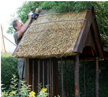
Andy Raffle completing the capping of the roof
